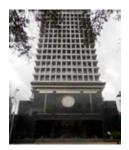
Richmond's current City Hall was constructed in 1970. By the late 1990s the structural integrity of the building was rapidly deteriorating. The culprit was its marble skin and in 2003 the facade was removed and the building re-skinned with a metal panel system.
