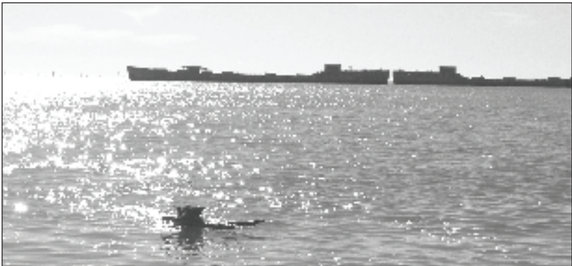
Concrete troop ships from World War II that have been placed in the Chesapeake Bay as a breakwater insure that the waters are always calm at Kiptopeke.
