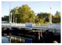
This single-leaf bascule bridge, one of the simplest and smallest of Maryland's movable spans, was built across the Pocomoke River in 1932. Carrying MD 12 into Snow Hill, it measures only 90 feet long, including the approach span. Its Neoclassical concrete tender's house is unoccupied; boaters must call in advance to schedule an opening.
