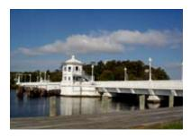
Erected in 1921, the Pocomoke City Bridge is one of only 20 movable bridges remaining in Maryland. It is of a type known as a double-leaf trunnion bascule movable bridge, the earliest type of movable bridge in the state. The Pocomoke City Bridge is notable for its decorative aspects and its intact bridge house at the draw.
