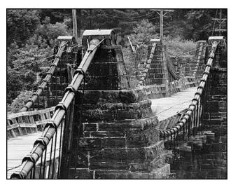
Suspension bridges are one of our oldest forms of bridgebuilding, dating back to the 1400s when Thangtong Gyalpo used iron chains to hang decks around Tibet and Bhutan. The first American iron chain bridge crossed Jacob's Creek in Westmoreland County, Pennsylvania in 1801. Cables consist-
