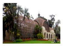
This unique structure raised for the 1915 Panama California International Exposition began with an iron frame salvaged from what was supposed to be a Santa Fe Railroad station. It was then skinned with over twelve miles of redwood laths to create one of the largest lattice structures in the world. The Botanical Building, and its Lily Pond out front, display a smorgasbord of over 2,000 permanent plants.
