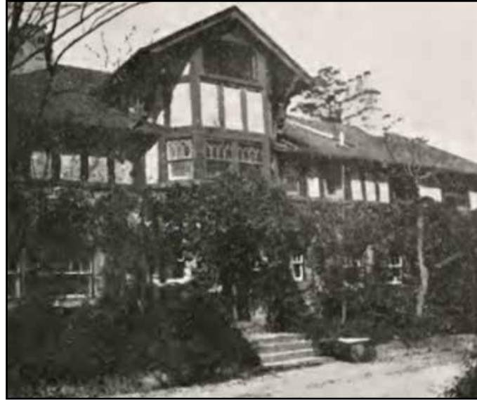
Lynncote, the original Erskine home in Lynn.
