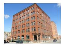
This six-story factory building from the early 1880s boasts a unique arched brick and steel construction that was designed to be not only fire-proof but earthquake-proof as well. The occupant then was the J.K. Hunt Paper Box Company, makers of "paper boxes of every description."
