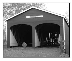
Covered bridges are the favorites of romantics everywhere. Wooden bridges were, however, the apogee of practicality - the roof protected the structural elements from the weather. It is estimated that over 14,000 covered transportation bridges have been constructed in the United States and fewer than 1,000 remain. Ohio is a prime hunt-
