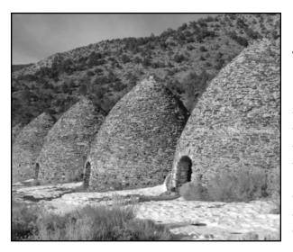
Beehive kilns were common structures in the early Western landscape. The kilns would burn timber into charcoal which was shoveled into smelters at mine sites to heat up and extract valuable metals from raw ore. Piñon pine converted into charcoal became 96% carbon and was the furnace fuel of choice since it burned more slowly than wood,
